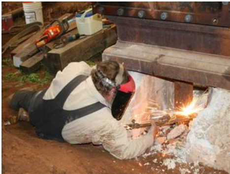
Upper left: Alan Hyatt cuts away pipes on the Globe engine for removal.
